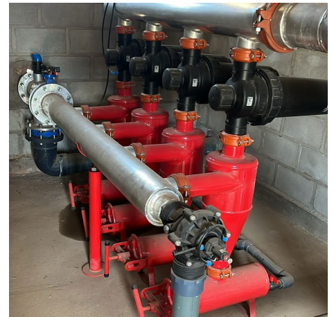
A co-operative water pump on loan to a grower
