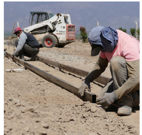
Pavements under construction at Los Pioneros Health Centre, Tilimuqui
